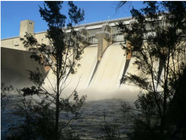
(A) General view of the dam spillway operation seen from the left bank (shutter speed: 1/800 s)
