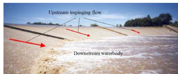
(A) Hydraulic jump at the toe of Chinchilla weir (Australia)
