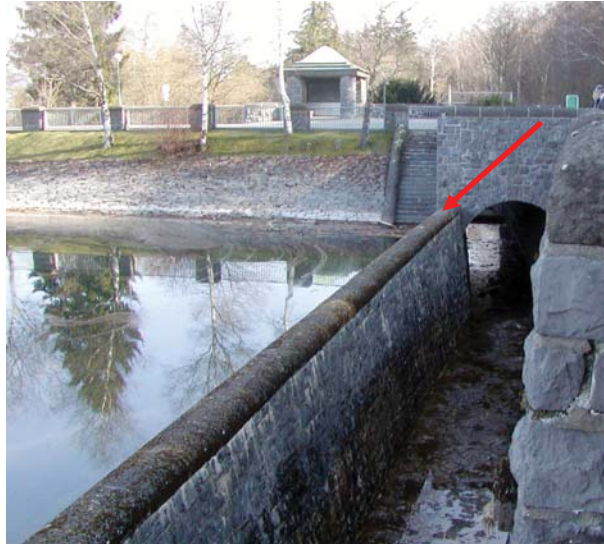
Figure 1. Half-round circular-crested weir at Sorpe Dam (Germany) on 31 March 2004.
