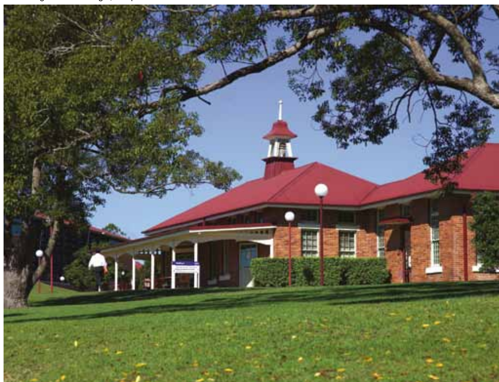
The heritage-listed Building 4, UQ Ipswich
