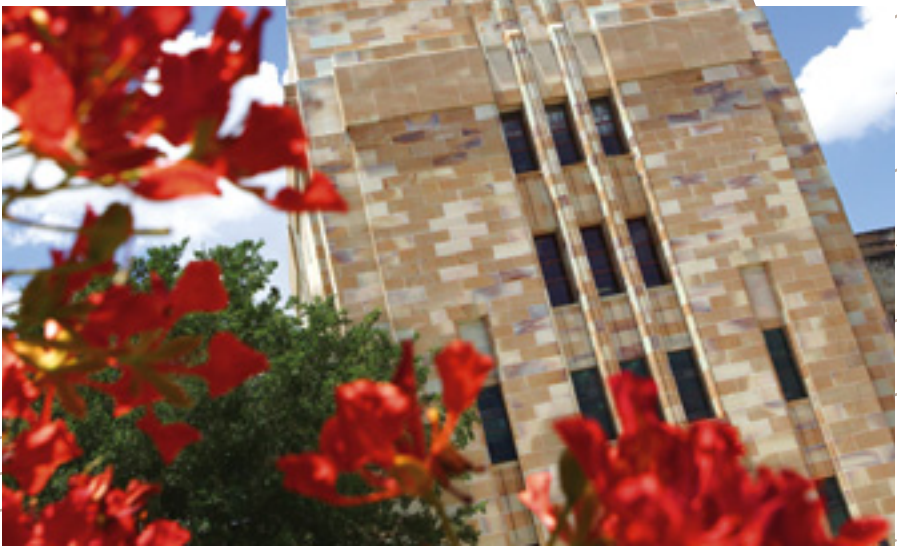
UQ's Forgan Smith Building at the St Lucia campus.
