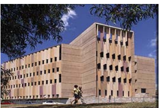
GPN Building at St Lucia Campus: The home of ACPACS and the ADR Program
