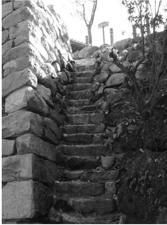
Fig. 1.1 (c) Storm waterway at Miya-jima (Japan) below Senjō-kaku wooden hall on 19 November 2001. The steep stepped chute ( \theta > 45^\circ , h \sim 0.4 m) was built during the 12th Century AD. The Senjō-kaku wooden hall was built by Kyomori (AD 1168) and left unfinished after his death.
