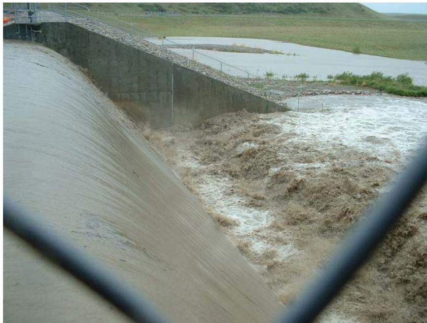
Hydraulic jump at the downstream of a steep spillway chute in Canada during a flood (Courtesy of John REMI)
